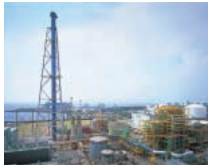
Power plant for Independent Power Producer
