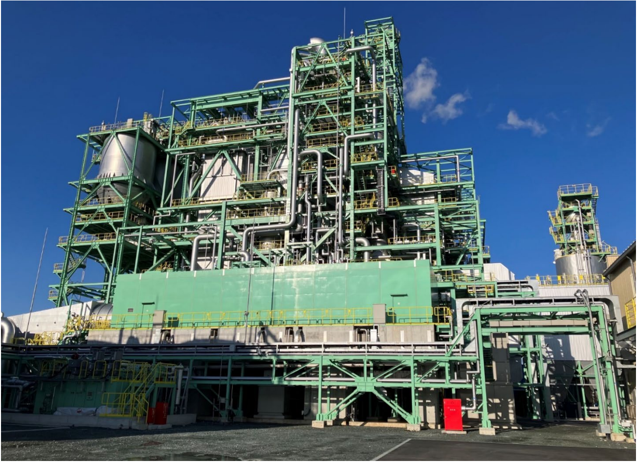
(Exterior of the Power Plant)
